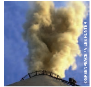
image Hatfield's Ferry Power Station, located near Masontown, Pennsylvania.
